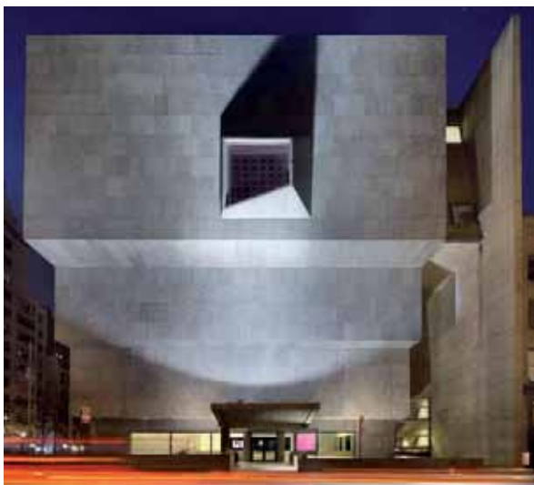
Dawna siedziba Whitney Museum przy Madison Avenue na Manhattanie, obecnie The Met Breuer Museum, fot. Ed Lederman, Metropolitan Museum of Art, https://www.inexhibit.com/wp-content/uploads/2016/03/The-Met-Breuer-facade-Madison-Avenue.jpg
