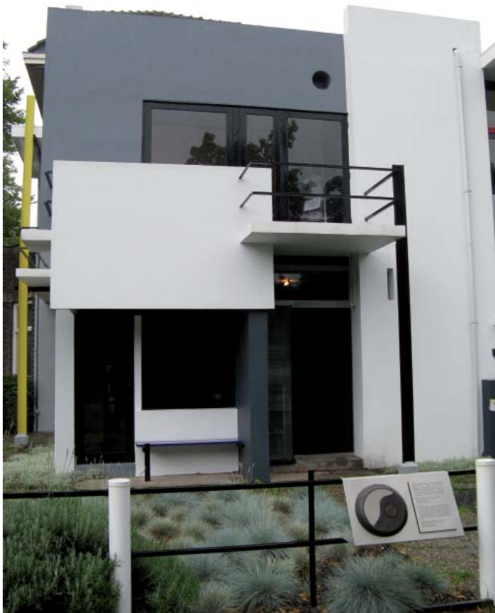
3. Rietveld Villa, fragment of the southern elevation
