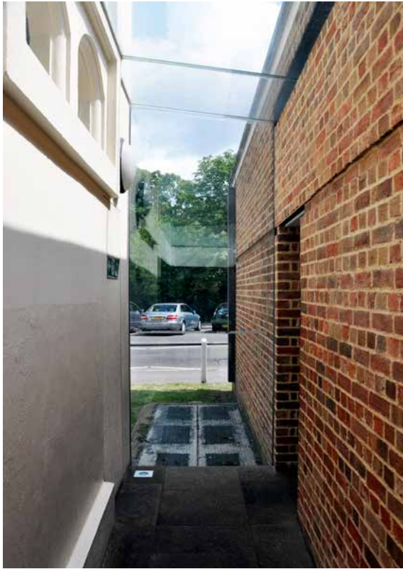
15. Glazed passage at the junction of the orphanage – the Almhouses (left) and a new entrance pavilion (right)
