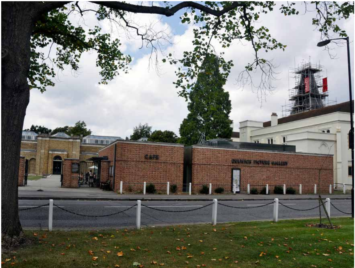
12. Dulwich Picture Gallery after enlargement, view from College Road, chapel's tower and buildings of the old orphanage to the right
